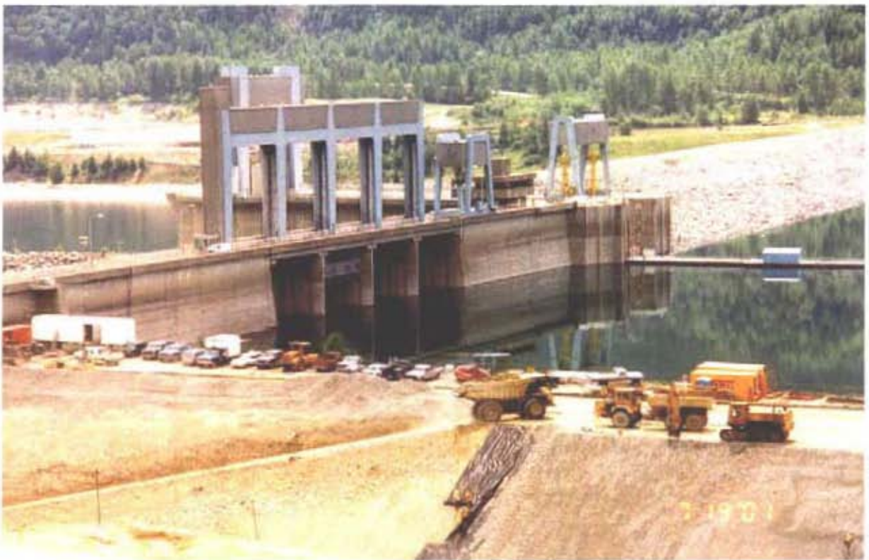
Figure 7: Upstream approach channel to the new powerhouse at Keenleyside Dam, July 2001.
