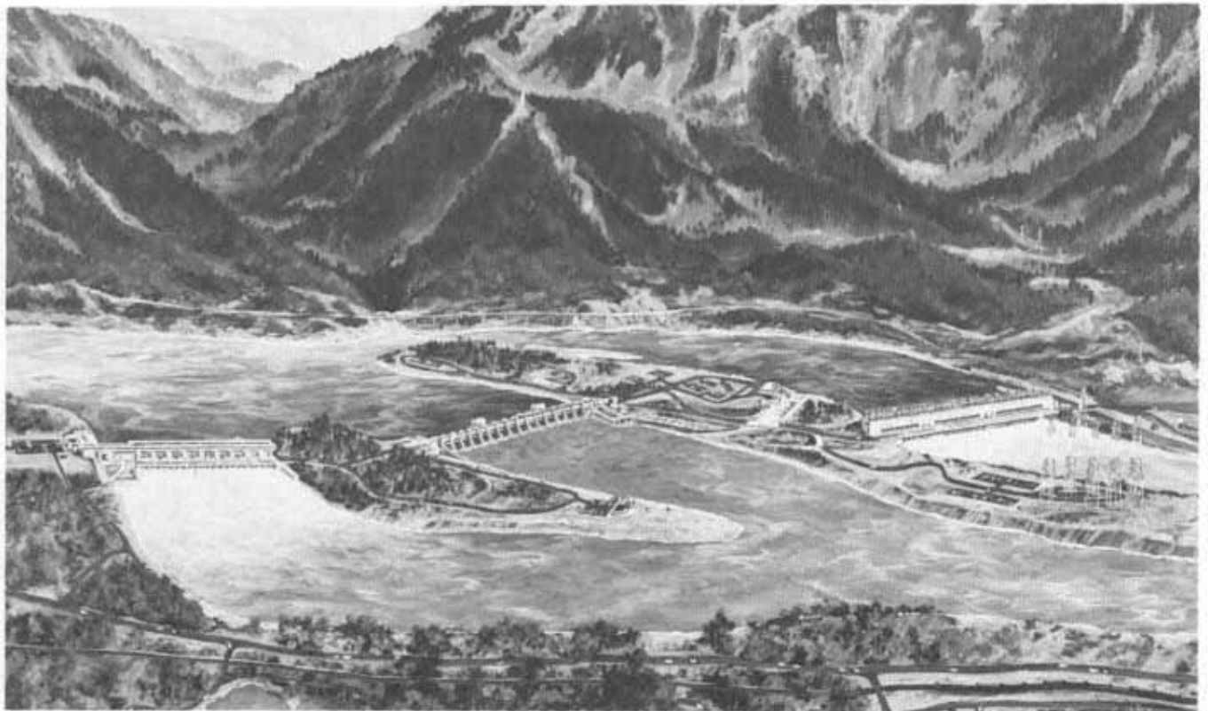
Looking downstream at Bonneville Dam second powerhouse construction on 16 July 1980 (above). Work was 87% complete on 31 July 1980. Power on line from the first of eight 66.5 MW units is expected in May 1981. Below is an artist's rendition of the completed project.
